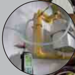
Testing the pressure regulator in the course of recording the measurement values over a defined period.
